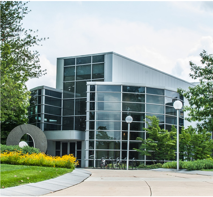
Top Photos (clock-wise): Front of the North Campus Research Complex, Building 18; Dr. Paul Lephart gives a tour of the new microbiology lab and automation line.
